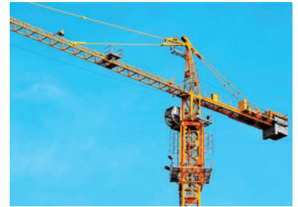
• 塔杆倾斜监测 Tower tilt monitoring
